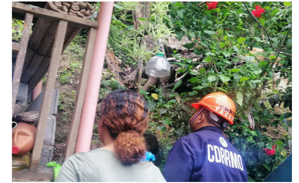
Inspection of landslide site
