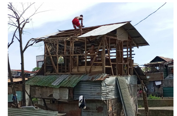
Clearing of illegal structures at Anibong
