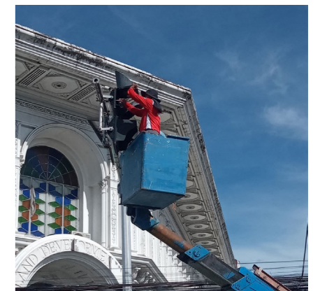
Repair of traffic lights
