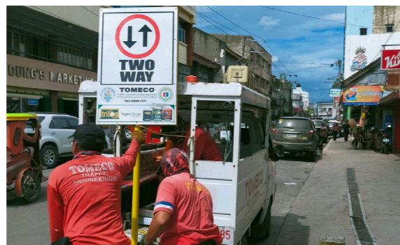
Installation of signboards
