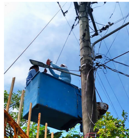
Repair of street lights
